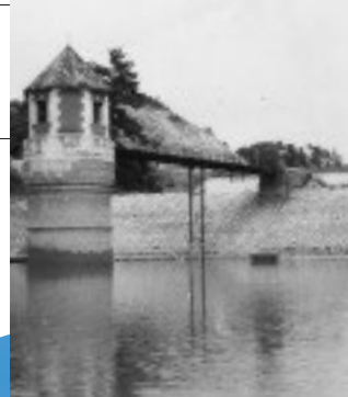
Old red brick intake tower
